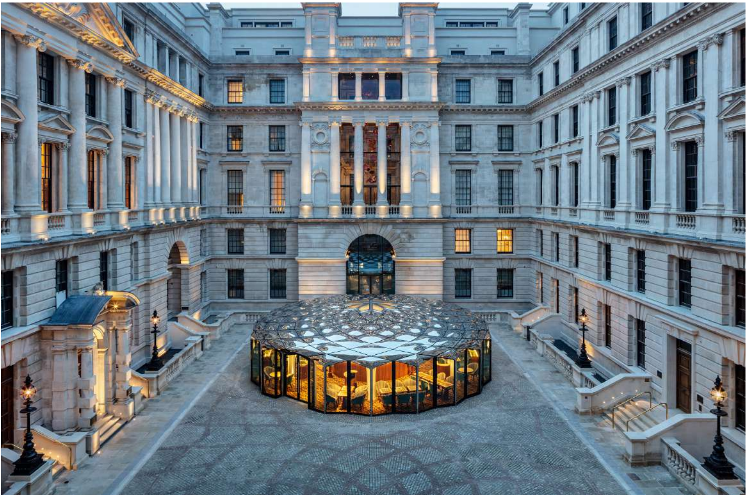
Front Picture: Restoration of the Farmyard at The Newt by Richard Parr, Photo by Rich Stapleton
